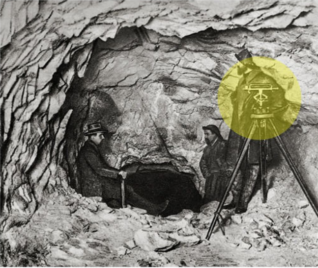
Figure 4. Surveyors with a level at the place of breakthrough (photograph in the archives of the Rhaetian Railway, Coire (Chur), reproduced with kind permission).
